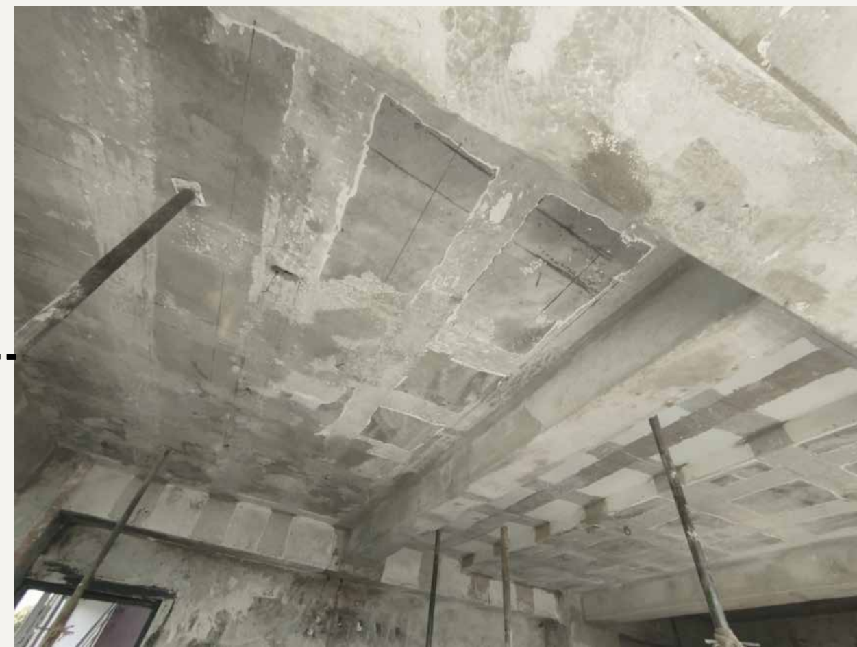
Surface preparation for Carbon fiber
