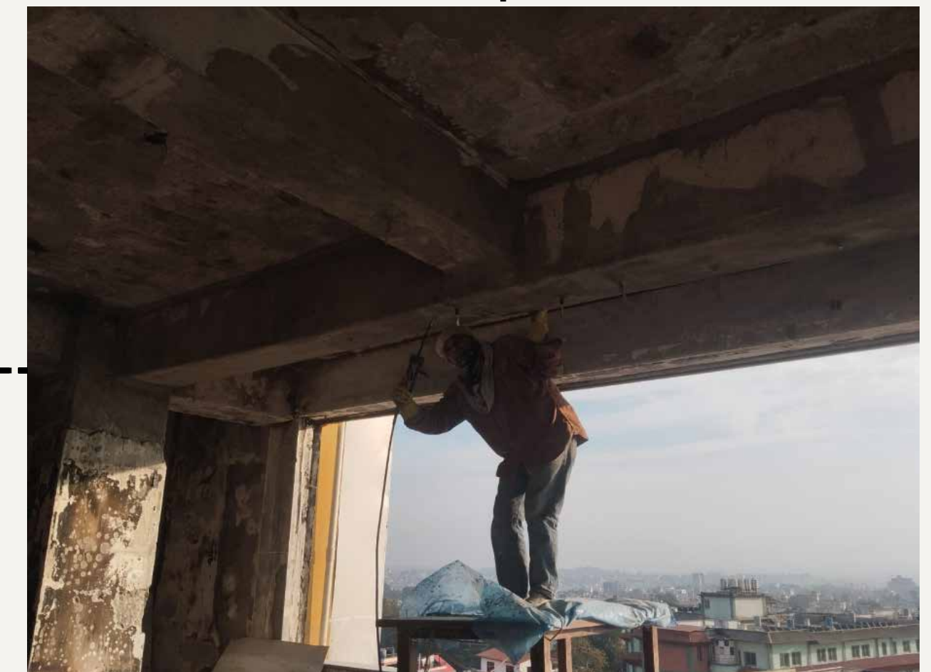
Pressure grouting
