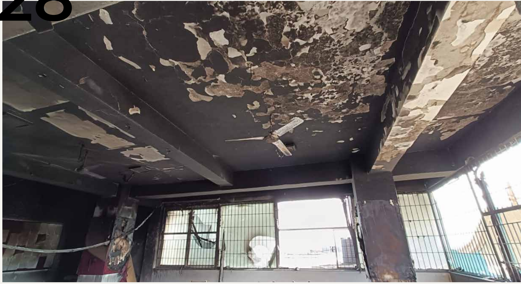
Fire damaged structure
